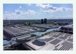
**18 MWp** that will make it possible to cover part of the needs of the exhibition site in Rho, while the remainder of the green energy generated will be fed into the grid. The project is a key pillar of Fiera Milano's Integrated Sustainability Plan 2024-2027, which aims to increase the use of renewable energy from 38% in 2023 to 70% in 2027 and which sees sustainability as a crucial element in attracting large touring exhibitions and driving business growth.
